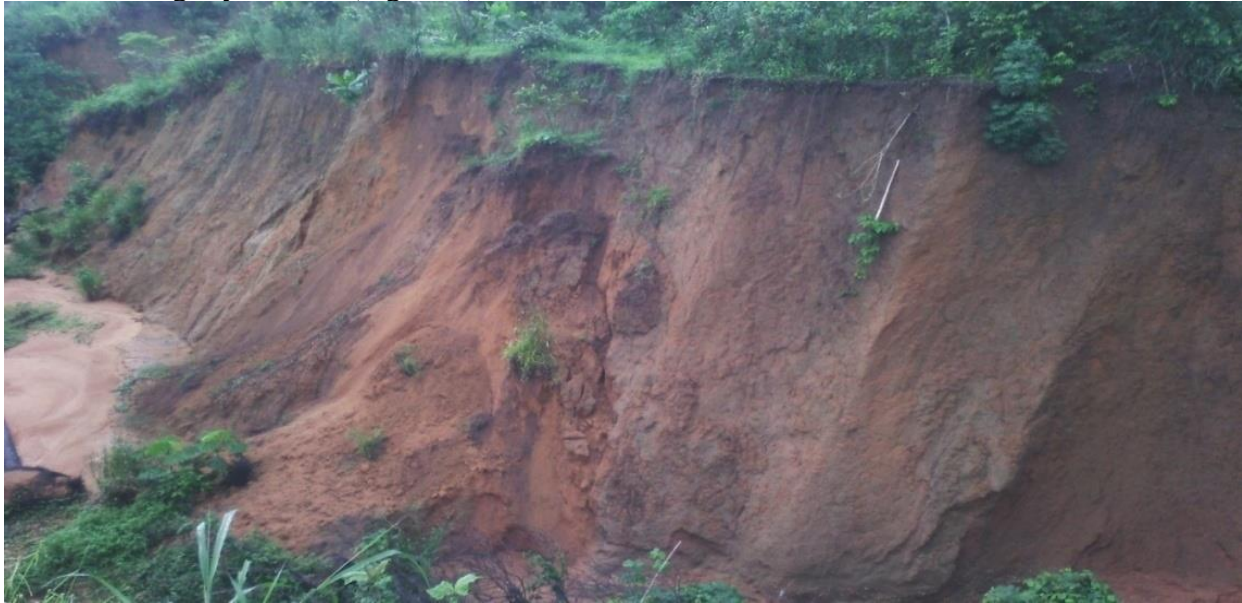
Figure 1: Gully erosion site in Uyo Source: Udoumoh et al. (2019)
